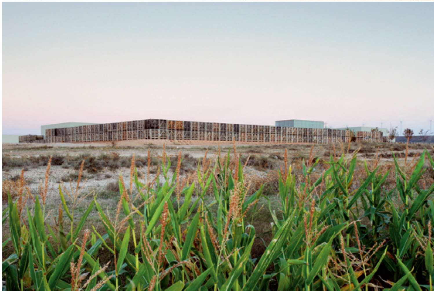
from top Turned into design features, elements such as reddish earth and large wood containers root the hotel into Navarre's local culture • Large, recycled wooden containers protect the site from the region's strong winds and extreme temperatures
